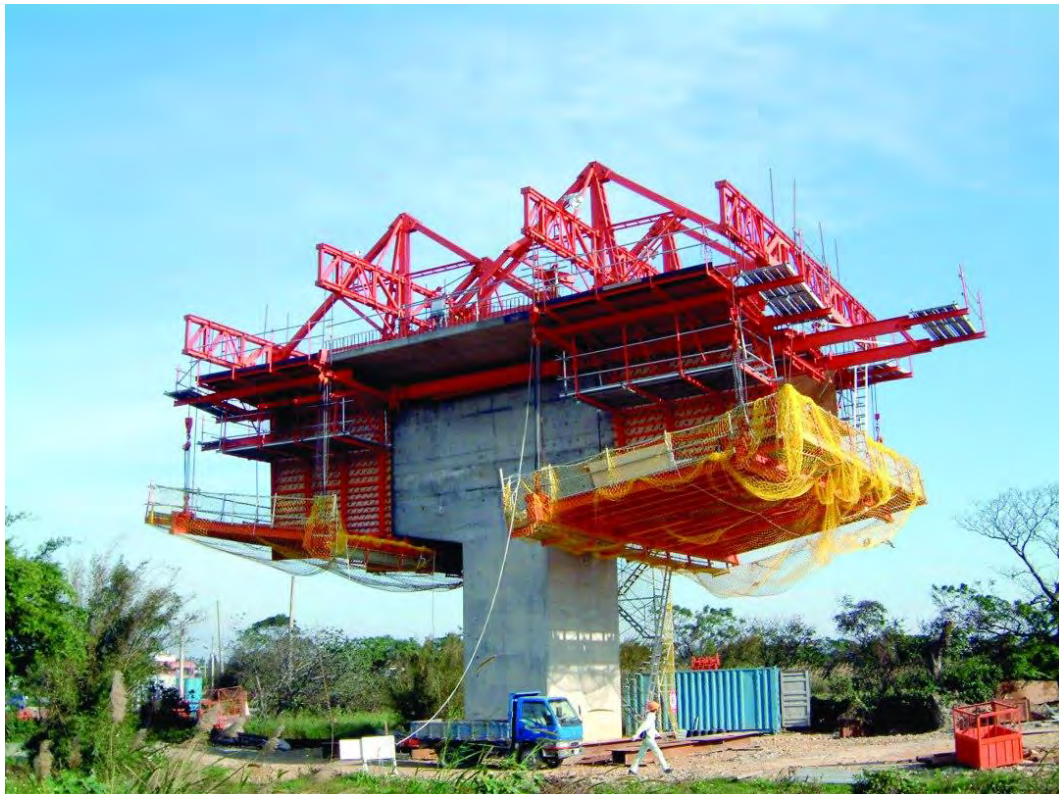
Figure 2.10: Travelling Formwork
